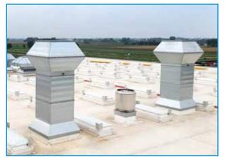
Intake hoods and deflector hoods in modular design. Both are manufactured according to the customer's request.
